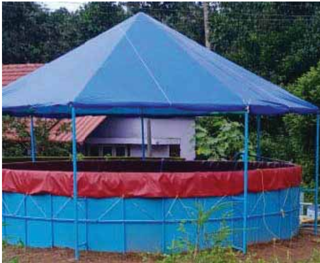
Fig. 2.12 Homestead tank constructed with GI sheet
